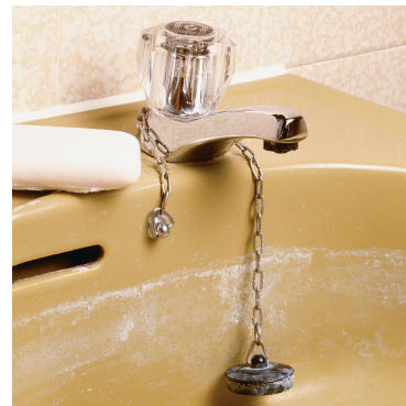
▲ The reaction of ions in hard water with soap produces a grey crud you can see after you drain the water.
